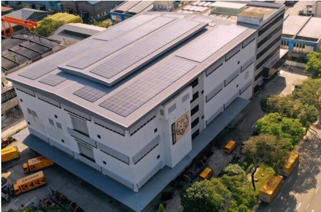
Starting with the largest building in our regional group, the Singapore office has been fully fitted with a solar roof comprising 665 panels covering 1,718 square metres. The solar energy generated is used to charge electric forklifts and power the air-conditioners in our warehouse and office. With this move alone, we have saved 196 tons of indirect carbon dioxide emissions.
